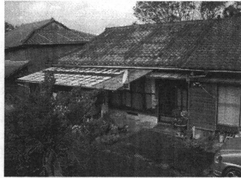
Figure10 Exterior of Case5
